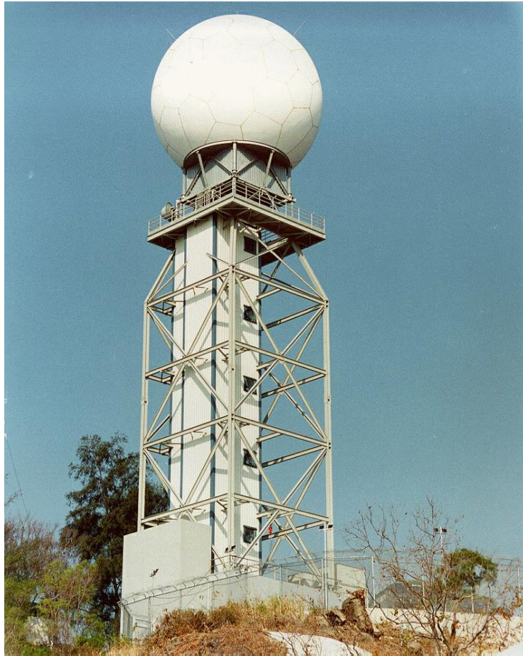
Figure A4-7. The terminal Doppler weather radar in Hong Kong
