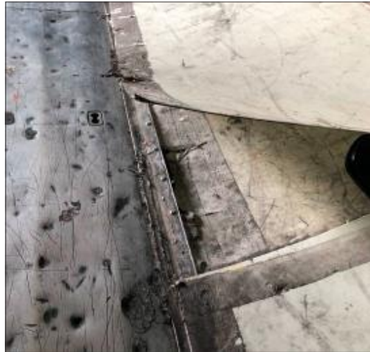
Figure 5-2. Damage to cargo compartment liners that can typically occur in service
