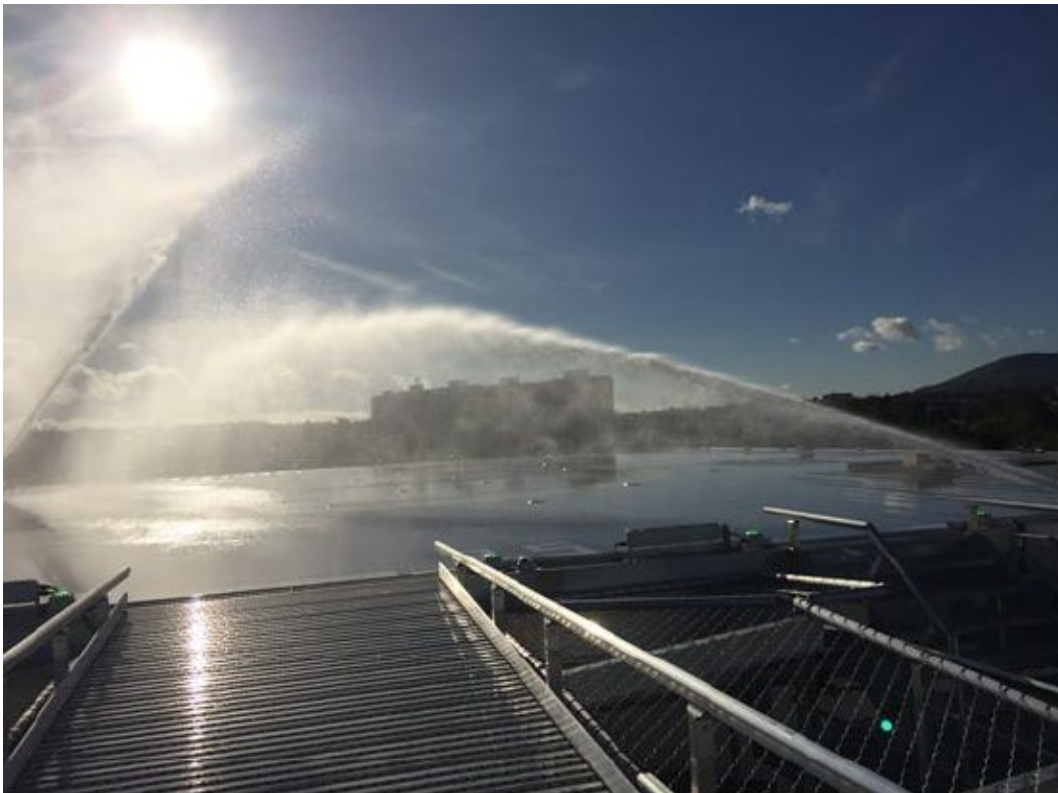
Figure II-6-3. Solid stream application utilising a fixed monitor system (FMS)
