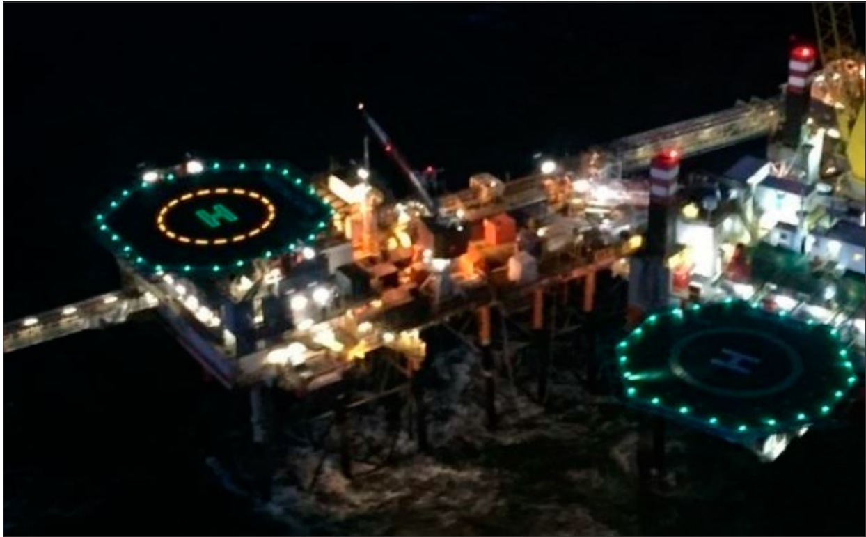
Figure I-5-13. Fixed platform (left) with the lit TD/PM and the lit heliport identification marking scheme. Mobile offshore drilling unit (right) with deck-mounted floodlighting system
