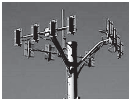
Figure U-1: A mobile telecommunications mast with three aerials – therefore three “sectors”
