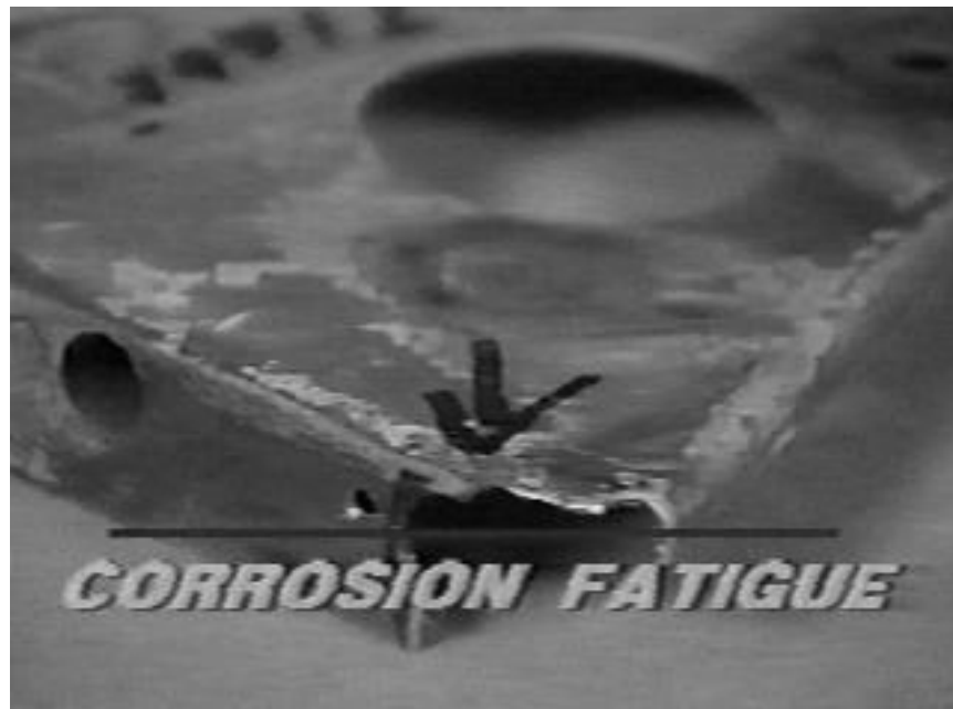
Figure III-9-75. Corrosion fatigue is the combined action of corrosion and the fatigue process on a metal.
