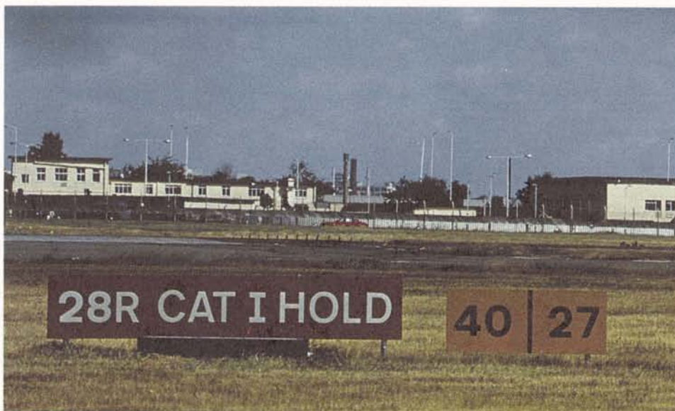
Figure A-2. A Category I holding position sign and an information sign located side by side
