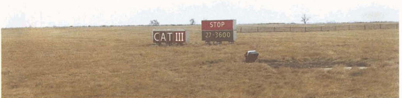
Figure A-4. A Category III taxi-holding position and a stop sign installed side by side
