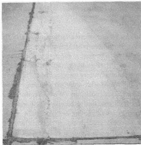
b. State of the damaged area after start of milling
