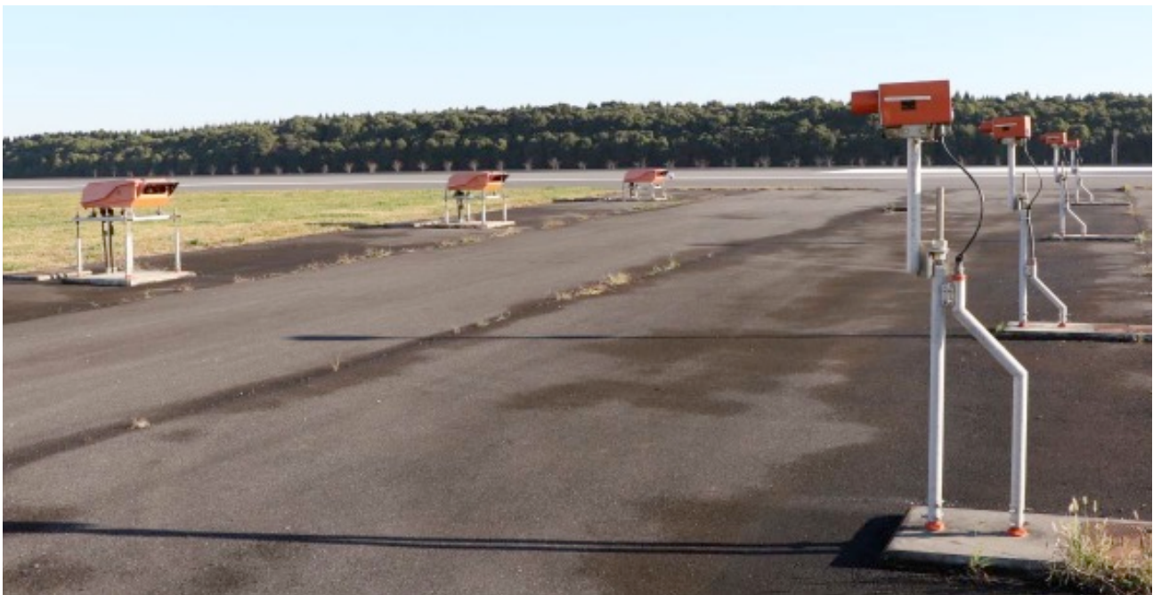
Figure 8-23. Installation of sensors for automatic monitoring Photo source: Narita International Airport
