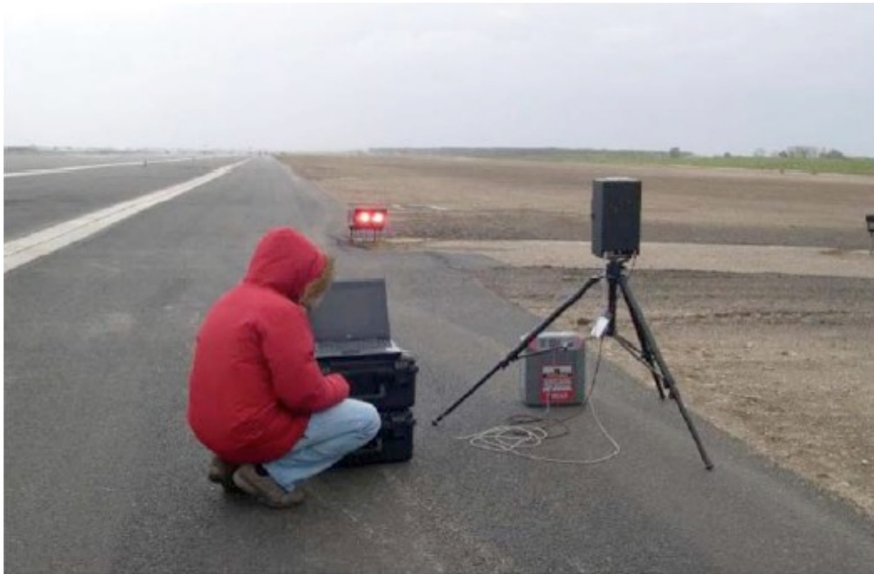
Figure 8-17. Typical set-up of image analysis method Photo source: Argos Ingegneria
