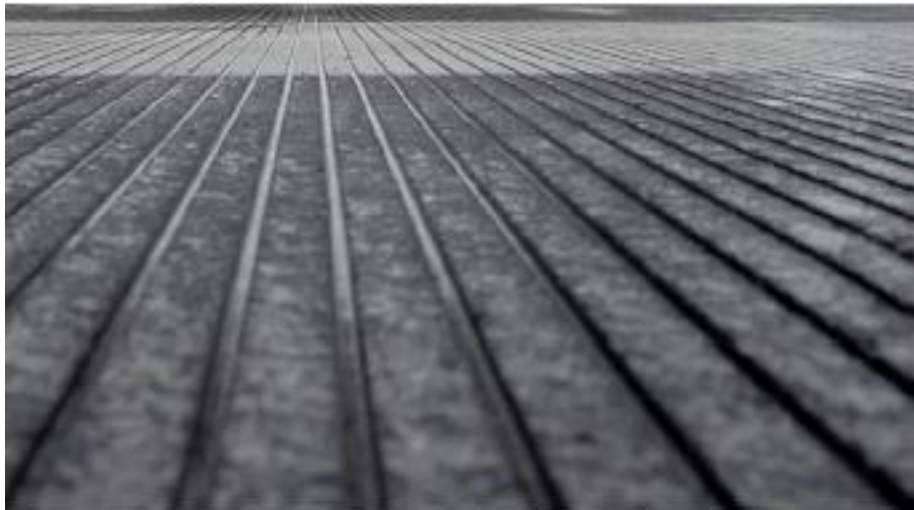
Figure A6-4. Grooving of asphalt surface (scale shows 2.5 cm divisions)
