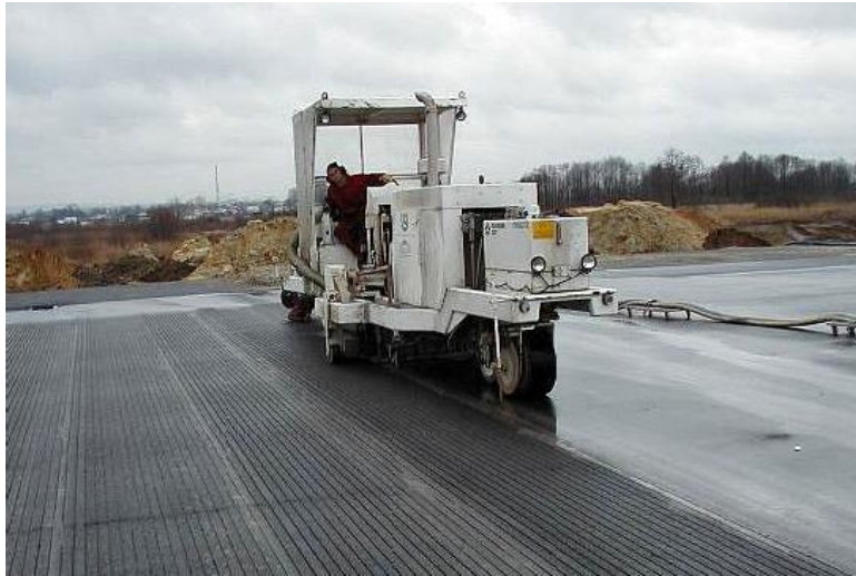
Figure A6-5. Grooving with saws
