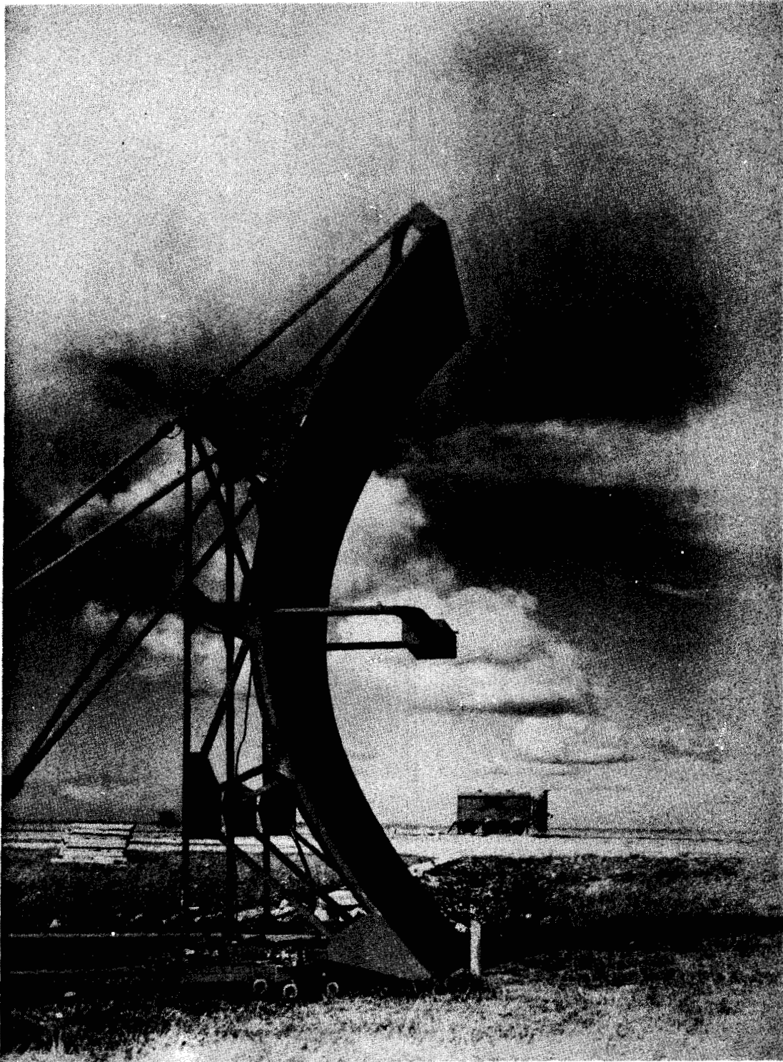
Fig. 8 - LOCALIZER ANTENNA (Remote from other antenna mounted on trailer)
