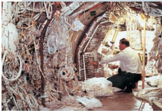
PUTTING IT ALL TOGETHER An engineer is seen working on the forward fuselage of the 002 Concorde prototype, in 1968. The 002 was the first Concorde assembled in Britain.
