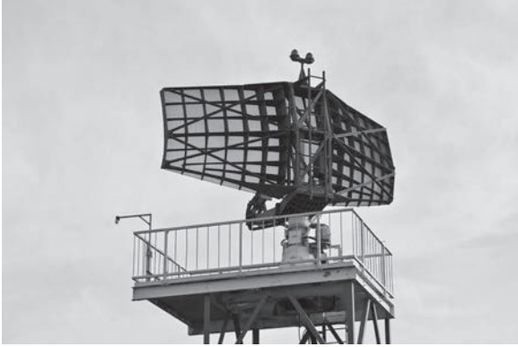
Figure 4.6a Radar tower (photo)
