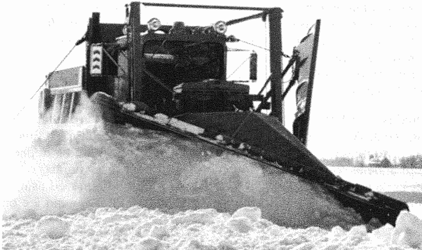
Figure 6-4. Snowplows move the snow to the pavement edges where snowblowers disperse the windrowed snow. (Photo courtesy FAA)
