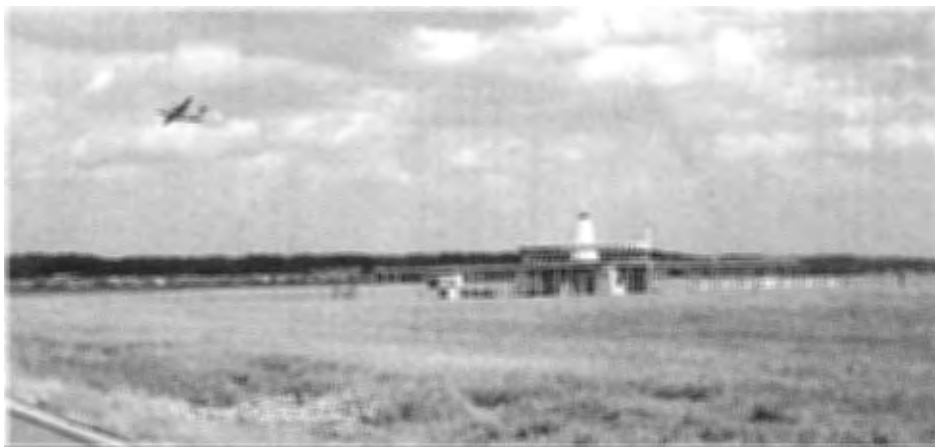
Figure 4-44. VOR beacon on the airfield at Washington Reagan National Airport. (Photo courtesy Seth Young)
