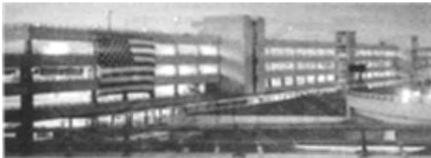
Figure 7-26. New multilevel parking garage at Washington Dulles International Airport. (Figure courtesy Metropolitan Washington Airports Authority)
