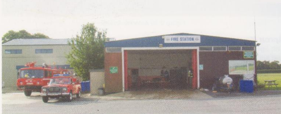
Figure 9.37 Fire Station at Kidlington, Oxon.
