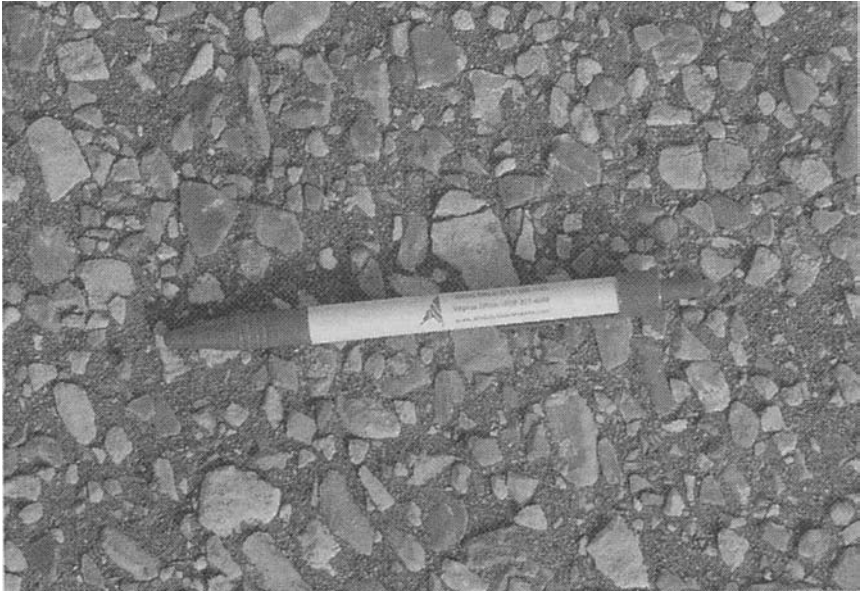
Figure D-11. Polished Aggregate.
