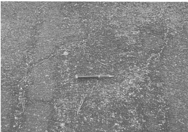
Figure B-19. Weathering and Raveling.
