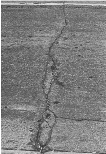
Figure B-8. Joint Reflection Cracking.
