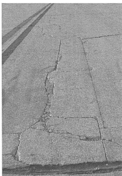
Figure E-7. Patching, Large.
