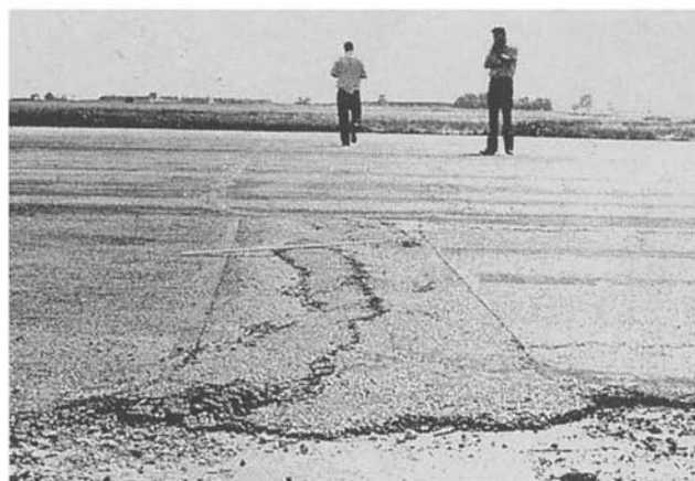
Figure D-10. Patching and Utility Cut Patch.
