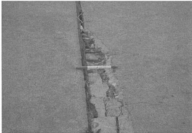
Figure C-19. Spalling, Joint.
