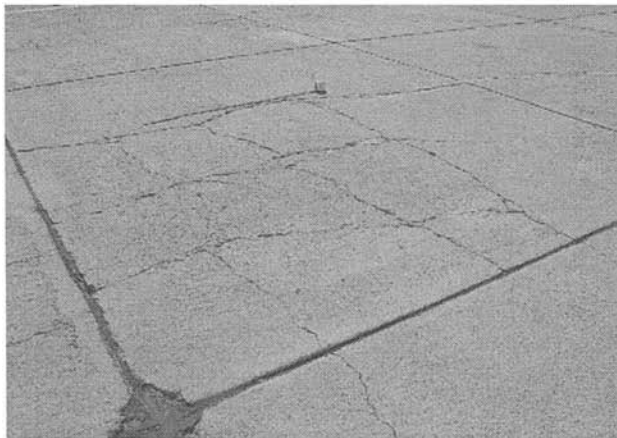
Figure E-12. Intersecting Cracks.
