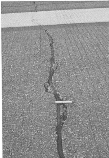
Figure D-8a. Longitudinal and Transverse Cracking.
