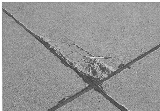
Figure E-6. Patching, Small.
