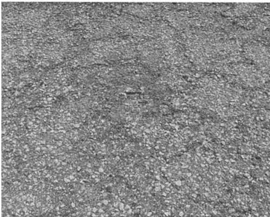
Figure D-12a. Raveling and Weathering.
