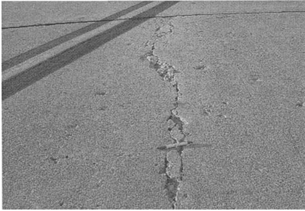
Figure E-3. Severity Crack.
