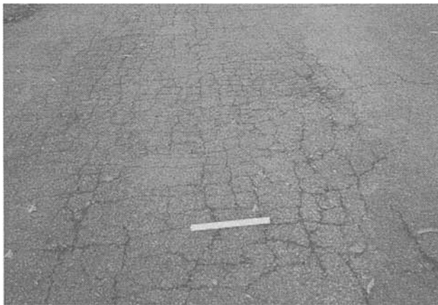
Figure B-1. Alligator Cracking.
