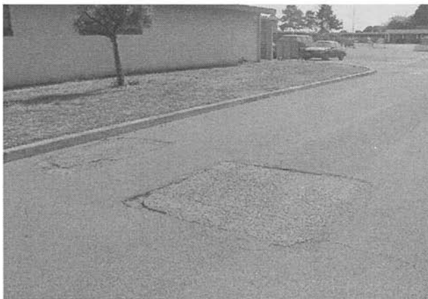
Figure B-11. Patching and Utility Cut Patching.
