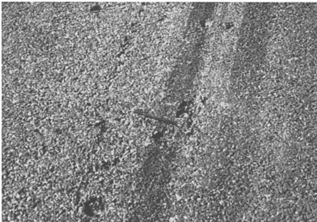
Figure D-12c. Raveling/Weathering on a Porous Friction Course Surface.
