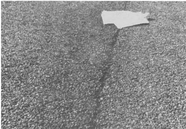
Figure D-8b. Crack in Porous Friction Course.
