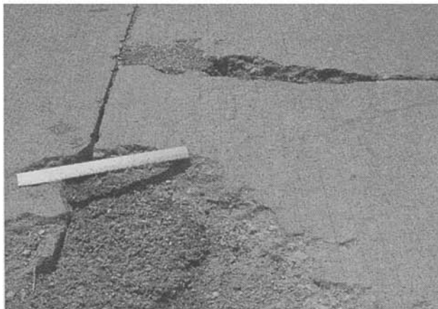
Figure C-18. Spalling, Corner.
