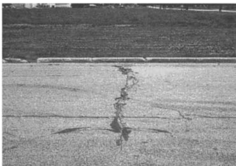
Figure B-10. Longitudinal and Transverse Cracking.
