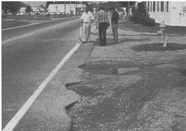
Figure B-7. Edge Cracking.
