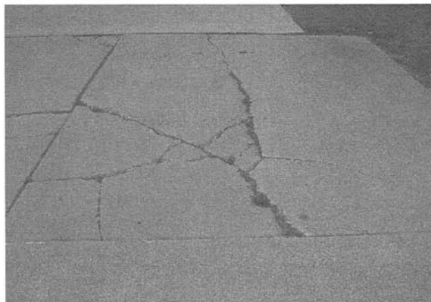
Figure C-3. Divided Slab.
