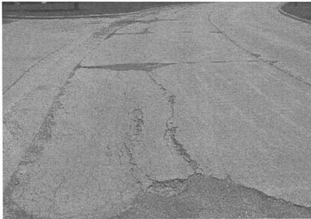
Figure C-4. Durability Cracking.
