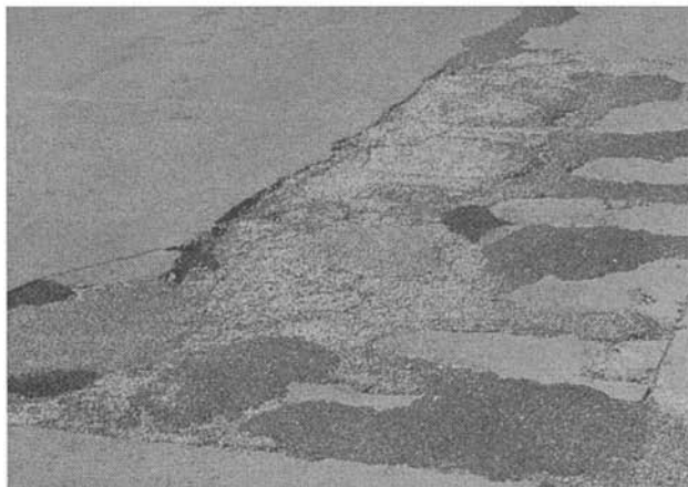
Figure C-16. Scaling, Map Cracking, and Cracking.
