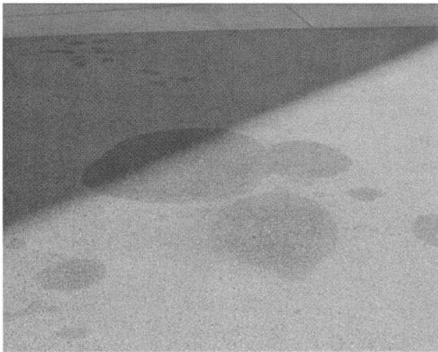
Figure D-9. Oil Spillage.
