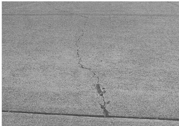
Figure E-3. Longitudinal Crack.
