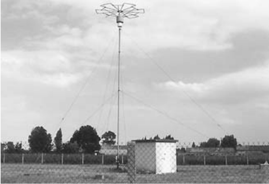
Figure 4-36. NDB nondirectional beacon. (Source: FAA)
