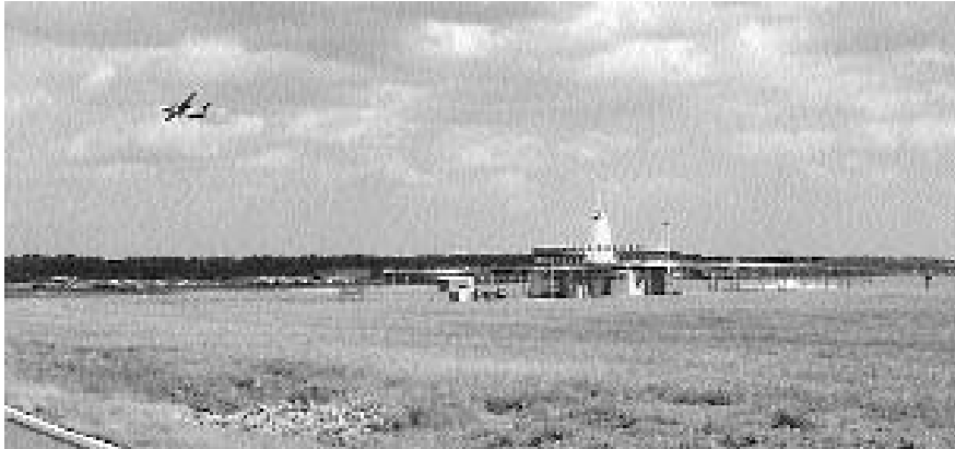
Figure 4-37. VOR beacon on the airfield at Washington Reagan National Airport. (Photo courtesy Seth Young)
