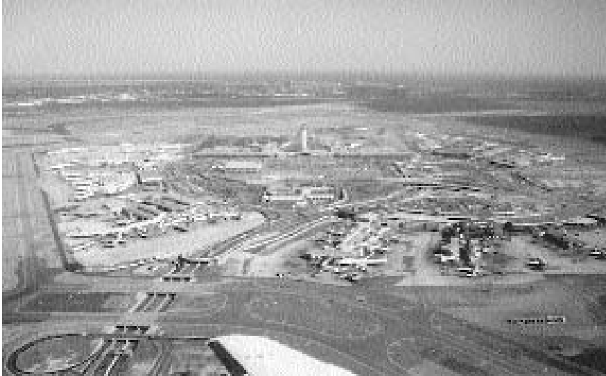
Figure 6-3. JFK International Airport in New York City provides an example of a multiple-unit terminal concept. (Source: www.airliners.net)
